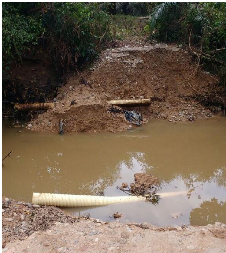
Figura 3. Dique #2 Colapsado
